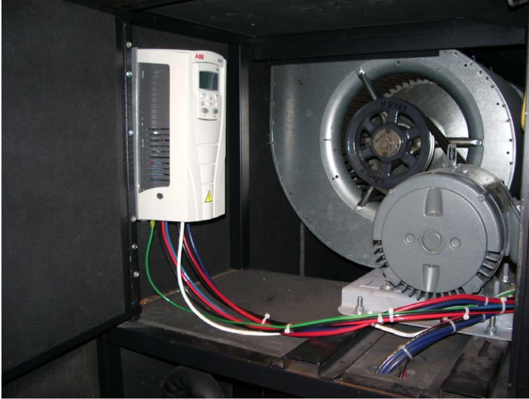
Figure 2. VSD installation: plain VSD mounted inside the CRAC (Credit: Symanski, 2012).
